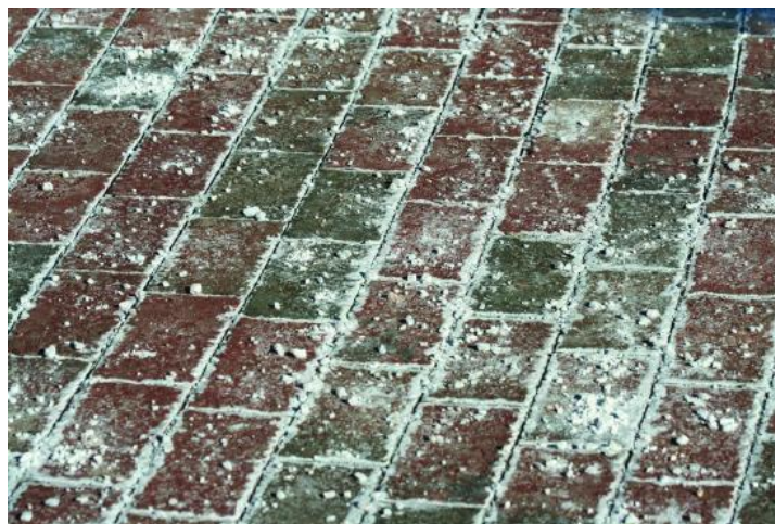
Figure 10.5.1: Salt and Safety © Thinkstock Salt or other compounds take advantage of the freezing point depression to minimize the formation of ice on sidewalks and roads, thus increasing safety.
